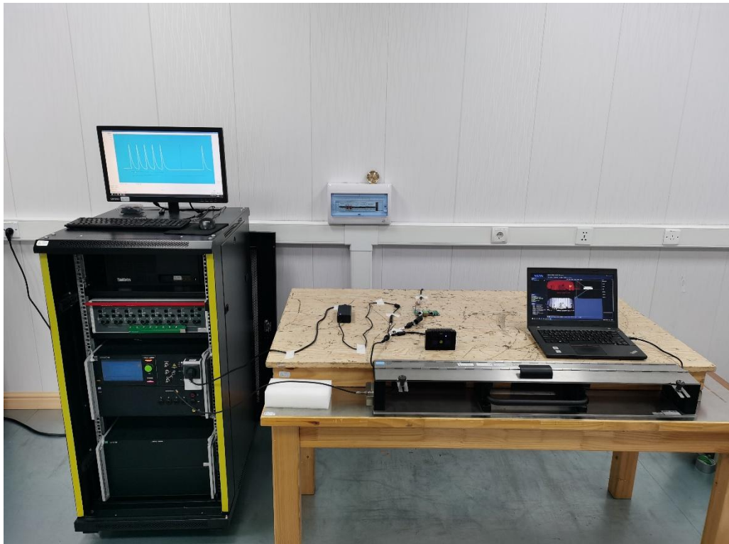
Wired network port
